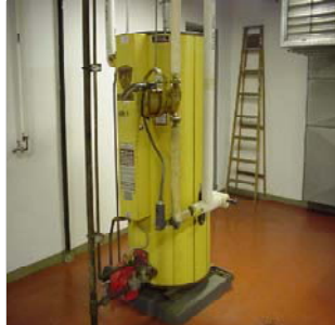
Rusted Domestic Hot Water Heater
